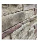
Many homeowners now choose the dry stack style of stonework, which is actually groutless. Mortar is used behind the stone to secure it in place, but there is no grout visible between the stones. This gives the work a very natural, casual appearance.
