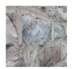
For a more old-world look. choose **overgrouting**. This technique uses a much heavier grout seam. Depending on the look you want, the grout can be even with or extend beyond the face of the stone, rather than being recessed like the standard
