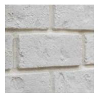
The most common grout technique is a standard or raked **joint**. This is what you typically see with brickwork, for example. The grout is evenly applied around the edge of each brick. When finished, the
