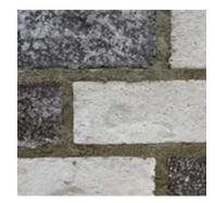
A **flush joint** is when a trowel is held flat against the brick and moved along the surface, so as to cut away the excess mortar. The resulting joint is flush with the brick.
