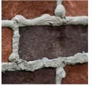
For a more oldworld look, choose overgrouting. This technique uses a much heavier grout seam. Depending on the look you want, the grout can be even with or extend beyond the face of the brick, rather than being
