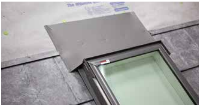
Fig. 31.3 - Backflash installed
