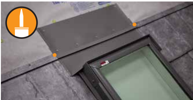
Fig. 31.4 - Backflash and Anchor Cleat installed
