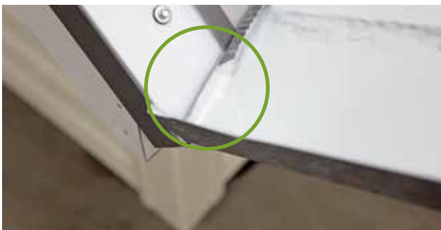
Fig. 19.4 - 2" drain slot in the first piece
