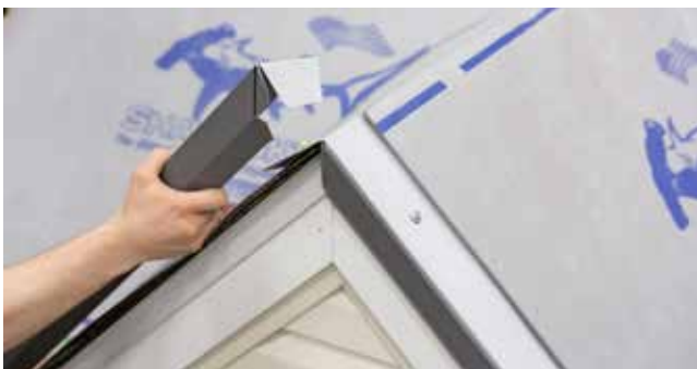
Fig. 15.3 - First piece at peak installed
