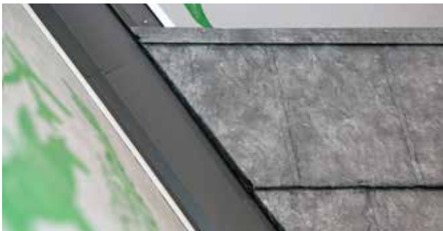
Fig. 21.4 - Panel installed into Valley
