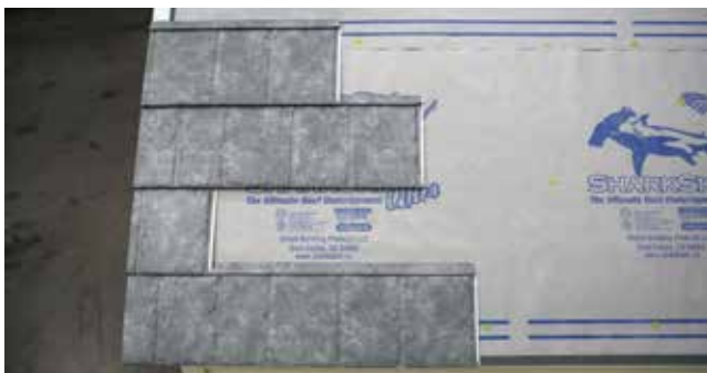
Fig. 19.3 - Slate profile starter pattern
