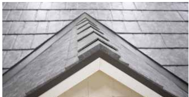
Fig. 34.4 - Ridge Cap installed
