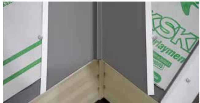
Fig. 16.3 - Valley flashing installed
