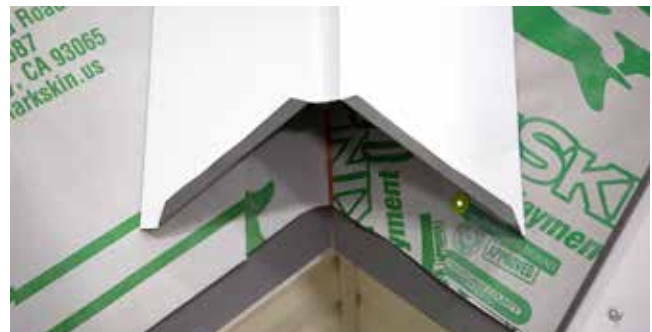
Fig. 16.2 - Valley flashing ready to install
