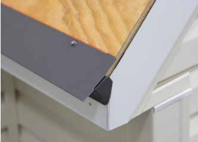
Fig. 11.1 - Outside corner piece installed
