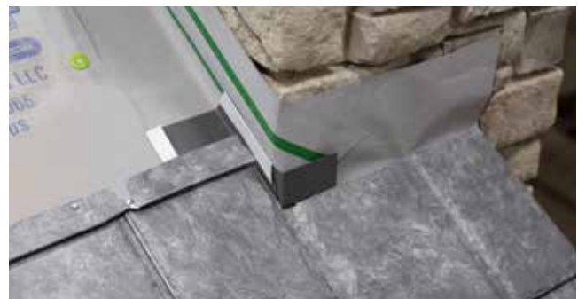
Fig. 26.3 - Panels installed over Underpan
