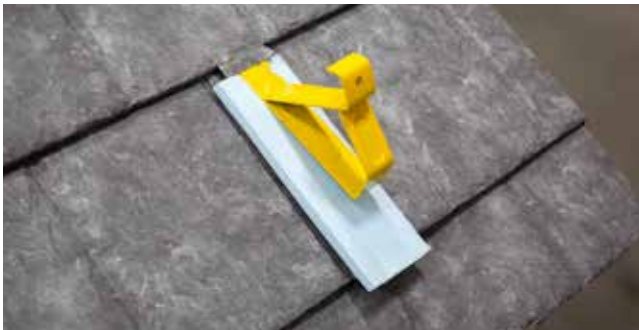
Fig. 9.2 - Nose of panel cut out
