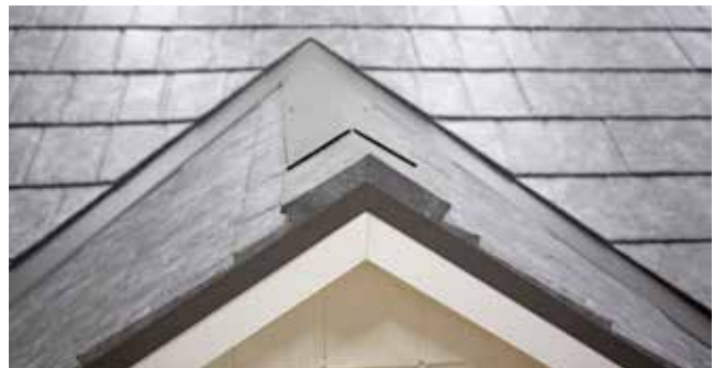
Fig. 34.3 - First Ridge Cap installed
