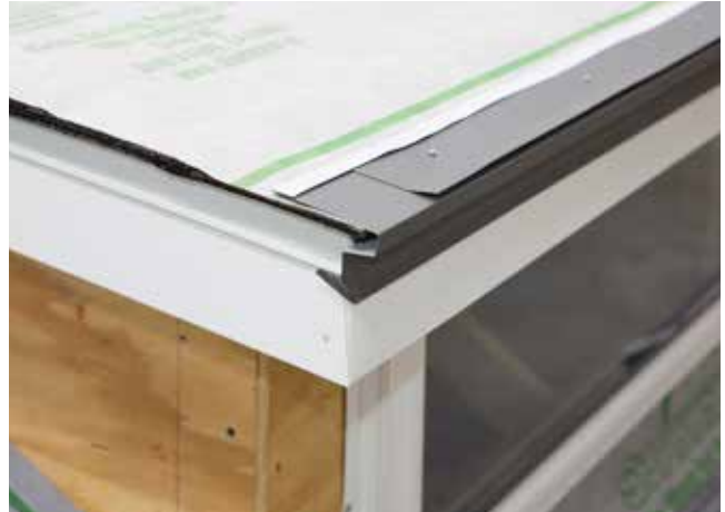
Fig. 14.1 - Outside corner piece installed
