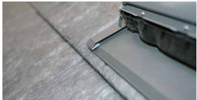
Fig. 30.4 - Open hem at bottom of sidewall
