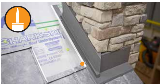
Fig. 27.3 - Sidewall installed at chimney
