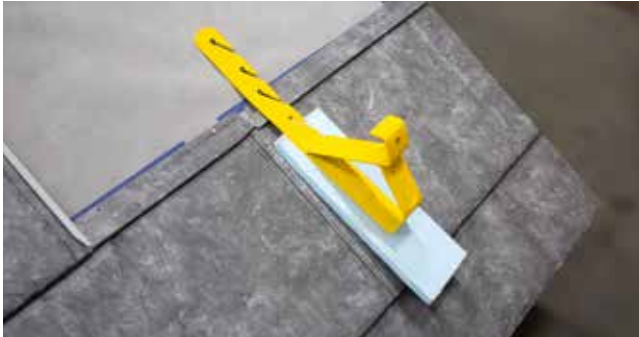
Fig. 9.1 - Roof jack installed
