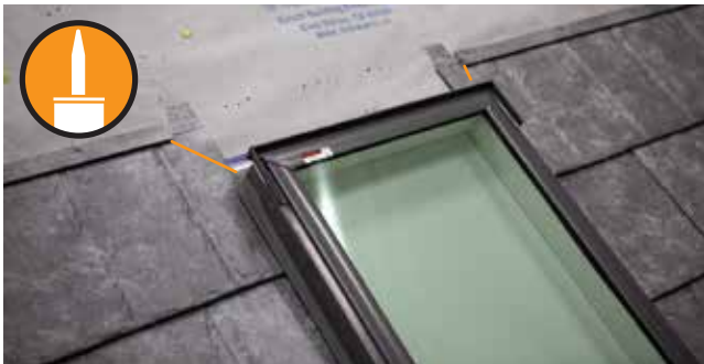
Fig. 31.2 - Panels installed and top lock opened
