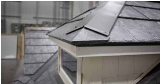
Fig. 33.3 - First Ridge Cap installed
