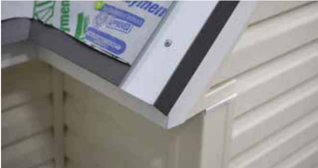
Fig. 13.1 - Outside corner piece installed
