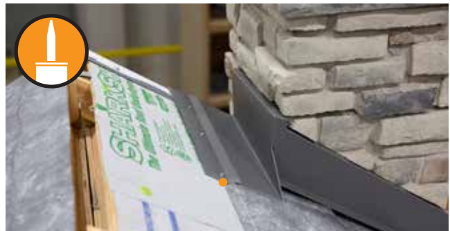
Fig. 28.4 - Backflash and cleat installed
