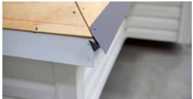
Fig. 12.3 - First outside corner piece installed
