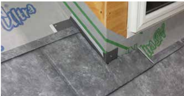
Fig. 25.4 - Panel installed over the Underpan
