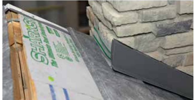
Fig. 28.1 - Panels installed beyond top of chimney
