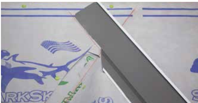
Fig. 17.2 - First piece of Valley flashing installed
