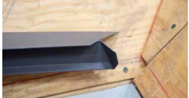
Fig. 12.1 - First inside corner piece ready to install
