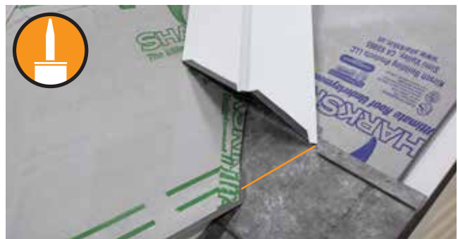
Fig. 18.3 - Valley flashing ready to install
