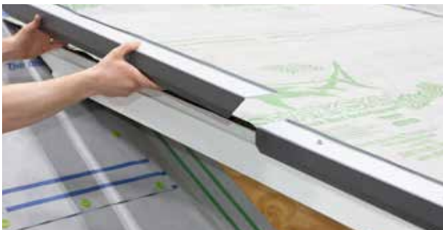
Fig. 15.2 - Overlap piece ready to install
