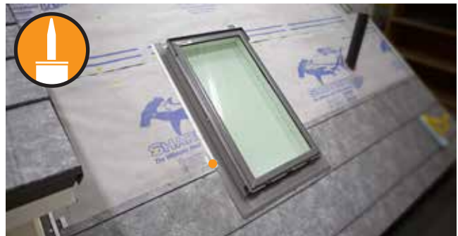
Fig. 30.3 - Sidewall installed at skylight
