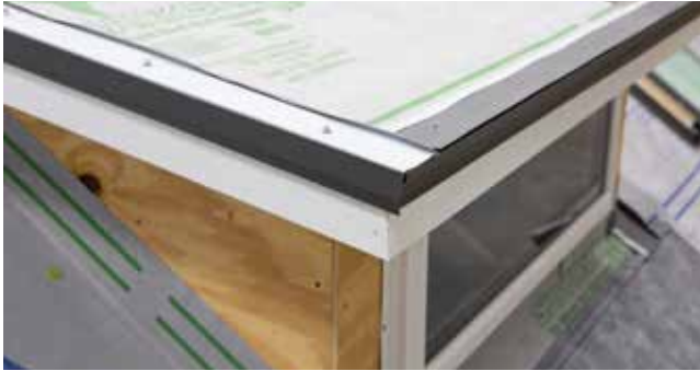
Fig. 15.1 - Outside corner piece installed
