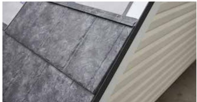
Fig. 20.3 - Panel installed into Rake Trim
