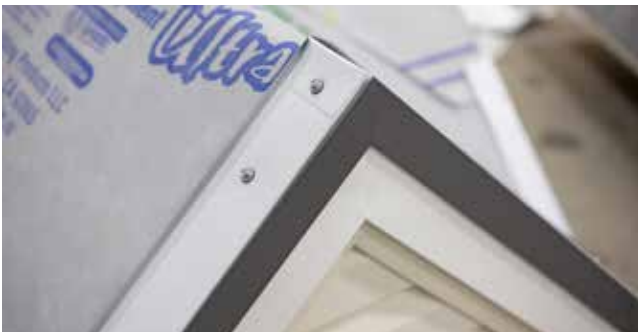
Fig. 13.4 - Second piece at peak installed
