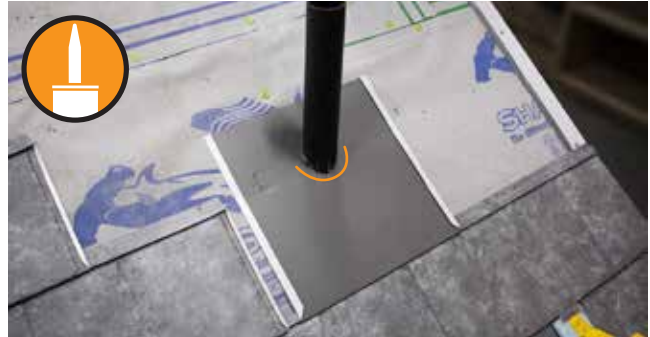
Fig. 32.1 - Underpan installed around vent pipe
