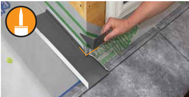
Fig. 25.2 - Underpan installed
