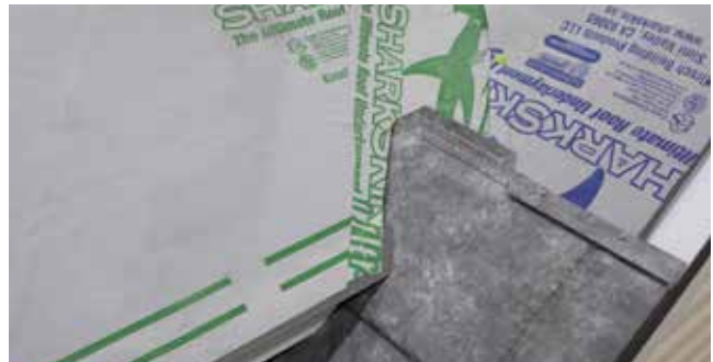
Fig. 18.2 - Top lock on last course of panel opened
