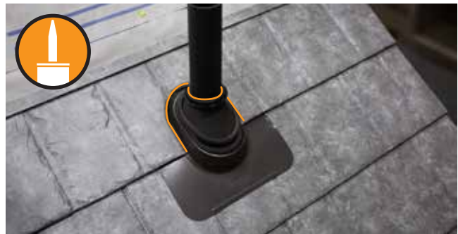
Fig. 32.4 - Panels installed around pipe flashing
