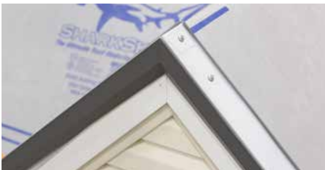
Fig. 15.4 - Second piece at peak installed
