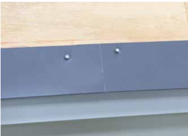
Fig. 11.3 - Overlap pieces installed
