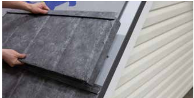
Fig. 20.2 - Panel ready to install
