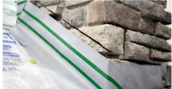
Fig. 26.1 - Chimney cut for Sidewall and Apron
