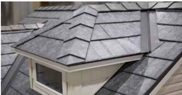
Fig. 33.4 - Ridge Cap installed
