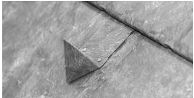
Fig. 35.2 - Panels installed over ProGrip diverter
