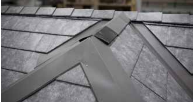
Fig. 33.1 - Hip Base installed
