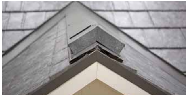
Fig. 34.2 - First Ridge Cap ready to install
