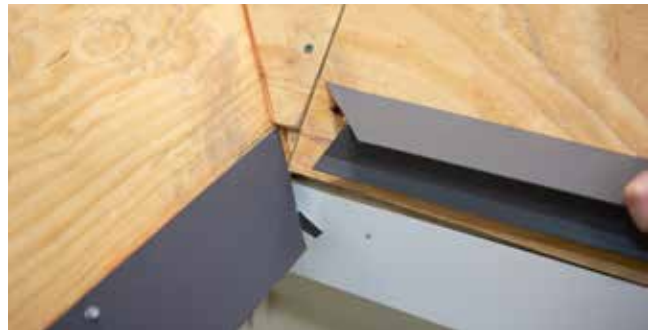
Fig. 12.2 - Second inside corner piece ready to install
