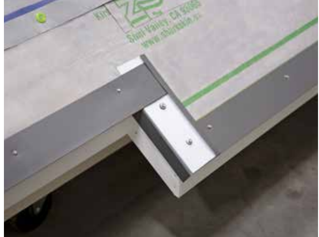
Fig. 24.1 - Short course with trims installed
