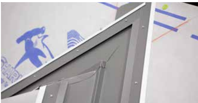
Fig. 17.4 - Valley flashings installed at ridge
