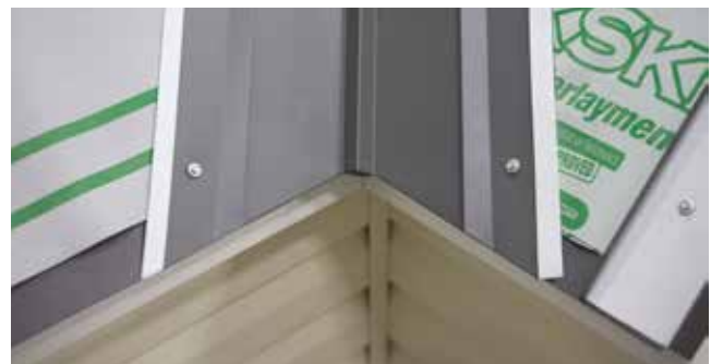
Fig. 16.4 - Anchor Cleat installed
