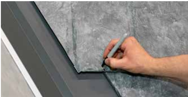
Fig. 21.2 - Panel positioned and ready to mark
