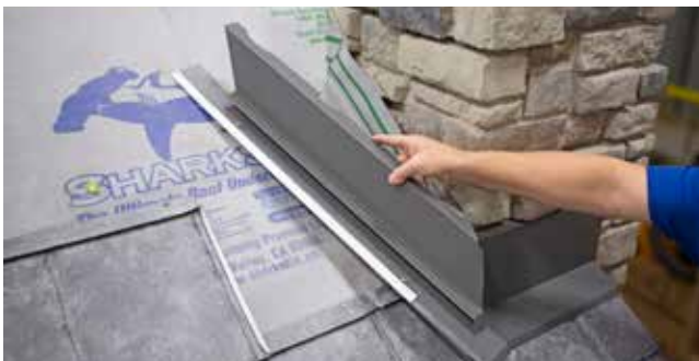
Fig. 27.2 - Sidewall ready to install
