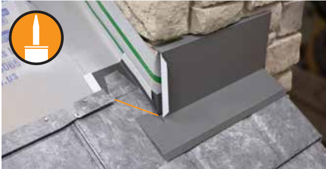
Fig. 27.1 - Top lock removed
