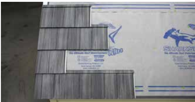
Fig. 19.2 - Shake profile starter pattern
