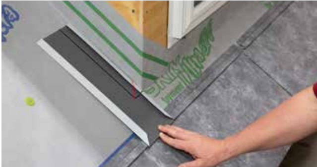
Fig. 25.1 - Underpan marked
