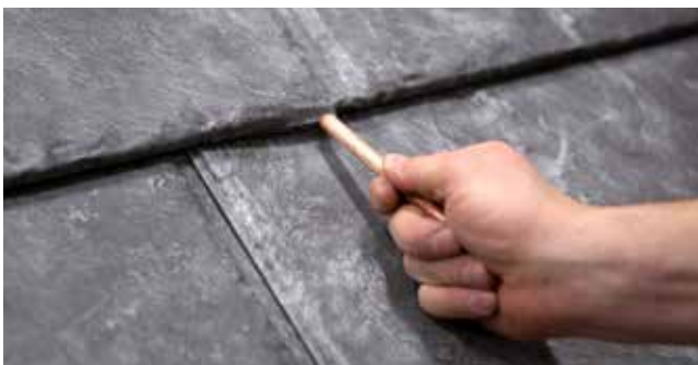
Fig. 9.4 - Nose of panel back in place
