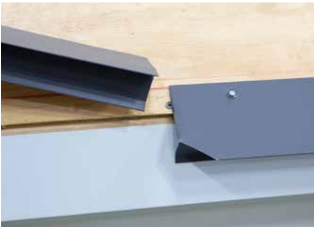
Fig. 11.2 - Overlap pieces cut and ready to install
