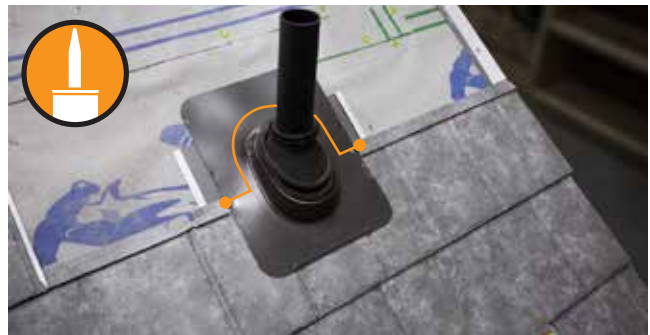
Fig. 32.3 - Pipe flashing installed over panels
