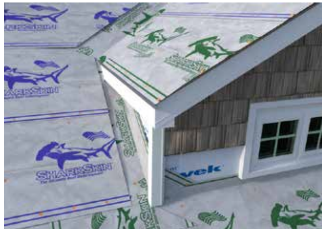
Fig. 10.2 - Ice and water (green) around skylight/dormer
