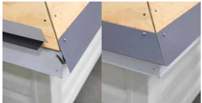
Fig. 12.4 - Second outside corner piece installed
